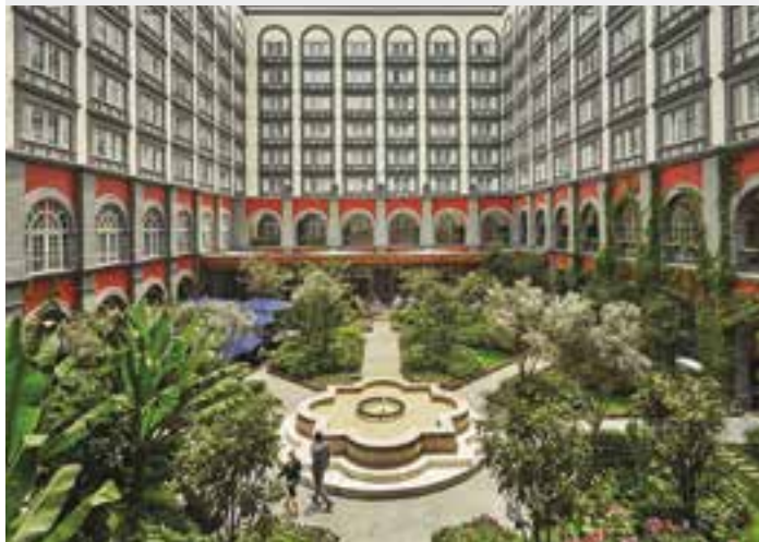
Four Seasons Hotel Mexico City Contemporary luxury hotel fronting the Paseo de la Reforma.
